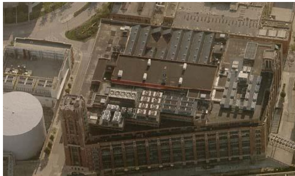
Fig.4.6. – Vista aérea do data centre Lakeside technology center, EUA [w18]
