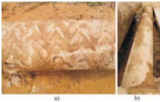
Figure 22 - Detail of pile shaft texture: a) bored; b) CFA (Costa Esteves, 2005).
