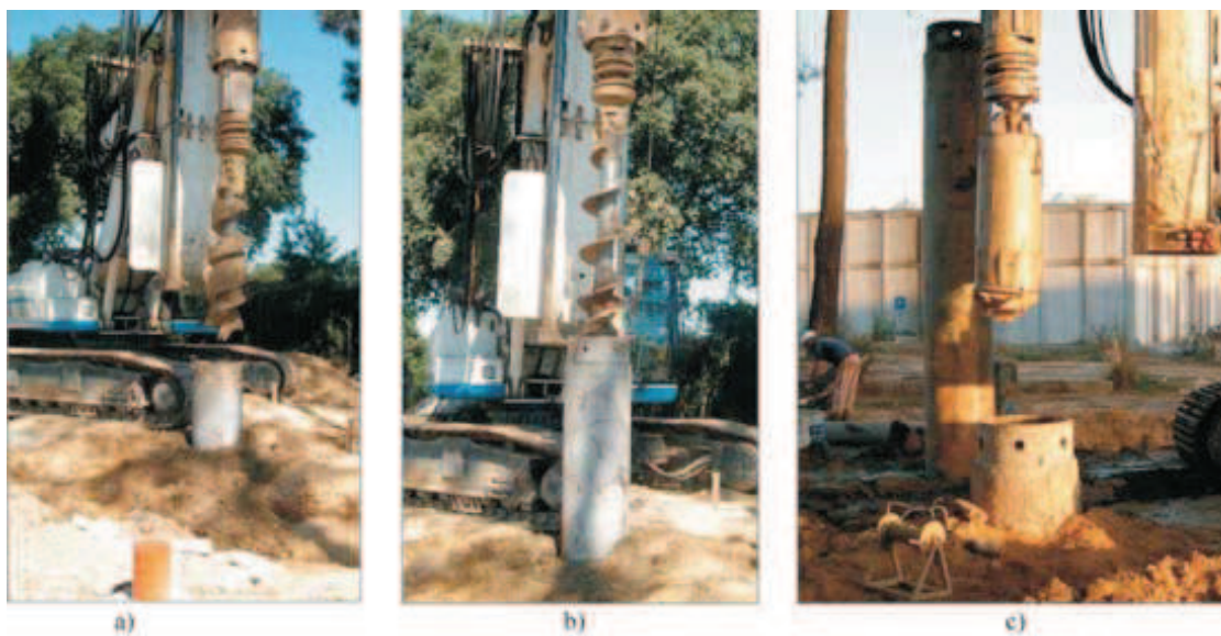
Figure 9 - Cleaning of the tube: a) and b) Borehole; c) Cleaning device (Costa Esteves, 2005).
