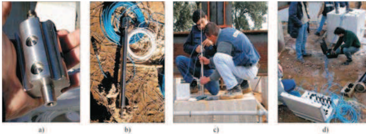
Figure 12 - Internal instrumentation: a) Anchor; b) Sensor c) Installation of sensors inside PVC tube; d) Sensors connections to reading unit (Costa Esteves, 2005).
