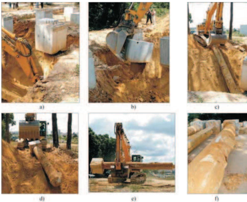
Figure 20 - Pile extraction (6 m): a) beginning of excavation; b) and c) and d) removal of pile from the soil; e) transportation of pile to the warehouse; f) general view of the pile after removal (Costa Esteves, 2005).
