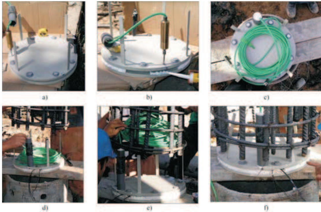
Figure 14 - Load cell installation (Costa Esteves, 2005).
