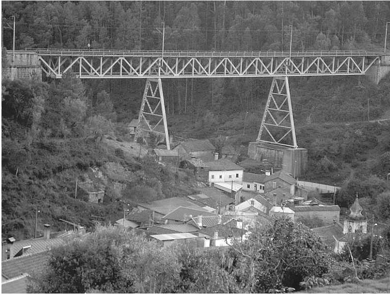
Figure 3.5 – Riveted metallic Trezói bridge.
