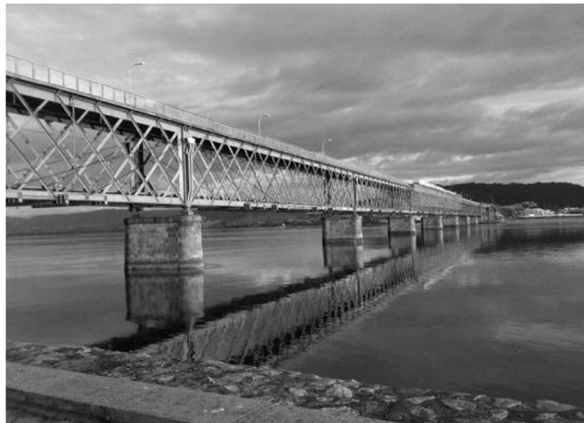
Figure 3.1 – Riveted metallic Eiffel bridge in Viana do Castelo.
