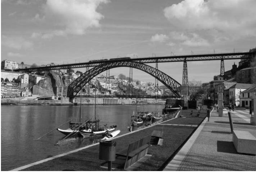
Figure 3.2 – Riveted metallic Luiz I bridge in Porto.
