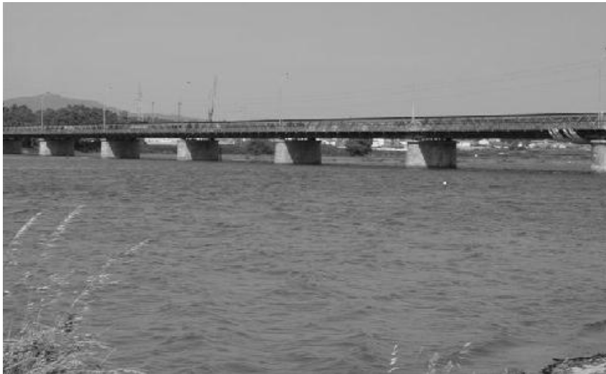
Figure 3.3 – Riveted metallic Fão bridge in Esposende.
