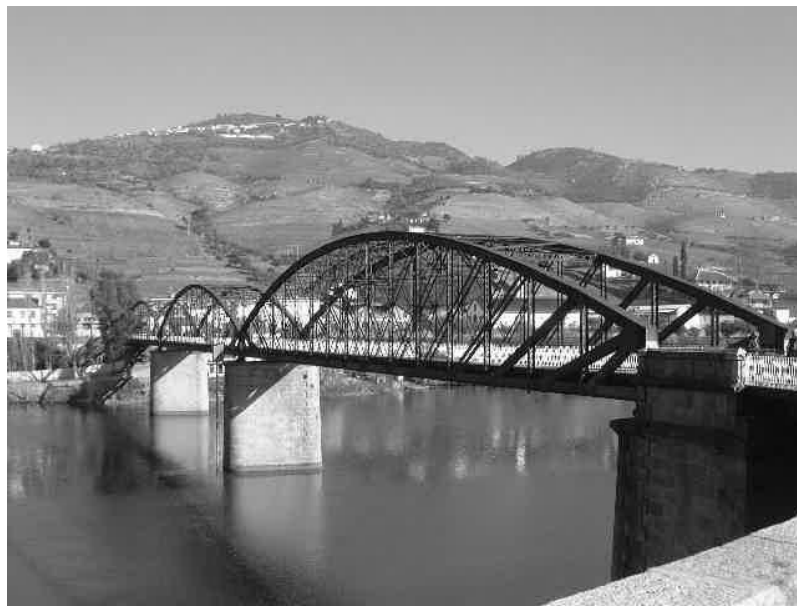
Figure 3.4 – Riveted metallic Pinhão bridge.
