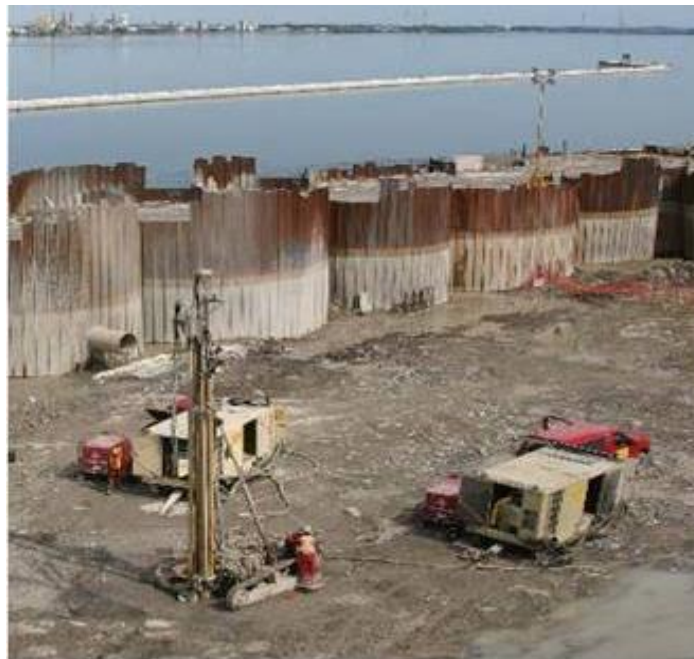
Fig. 1. 3 - Ensecadeira de células (Sir Adam Beck Power Station - Niagara Falls, Ontario) [5]
