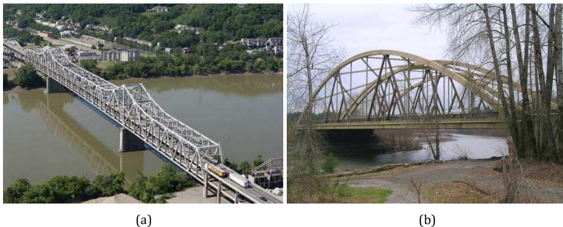
Figure 8.2 – Tested bridges (II): (a) Brent-Spence Bridge, USA (Harik et al. , 1997); (b) Toutle River Bridge, Washington, USA (Roeder et al. , 2000).
