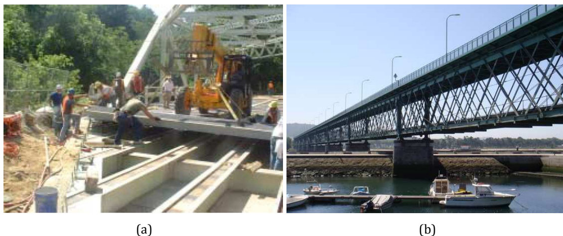
Figure 4.3 - (a) Placement of a new FRP composite deck on a truss bridge (Fu et al. , 2007); (b) double-deck steel truss bridge monitored by means of fiber Bragg grating sensors.
