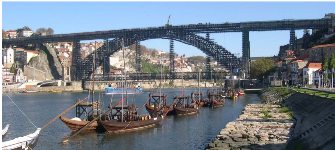
Figure 7.5 – View of Luiz I Bridge during the rehabilitation works.
