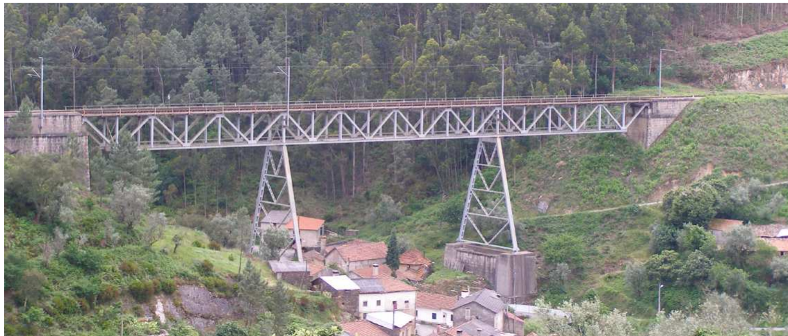
Figure 2.1 - General view of Trezói Bridge.
