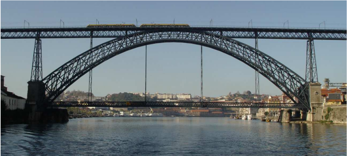
Figure 6.1 - Luiz I Bridge.
