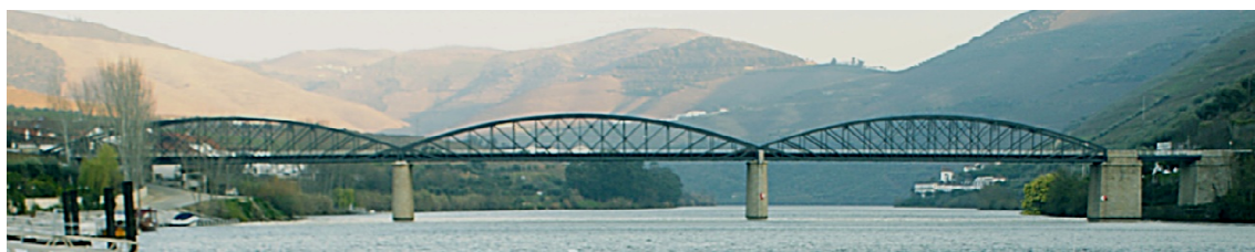
Figure 3.1 - Pinhão road bridge over the Douro river.
