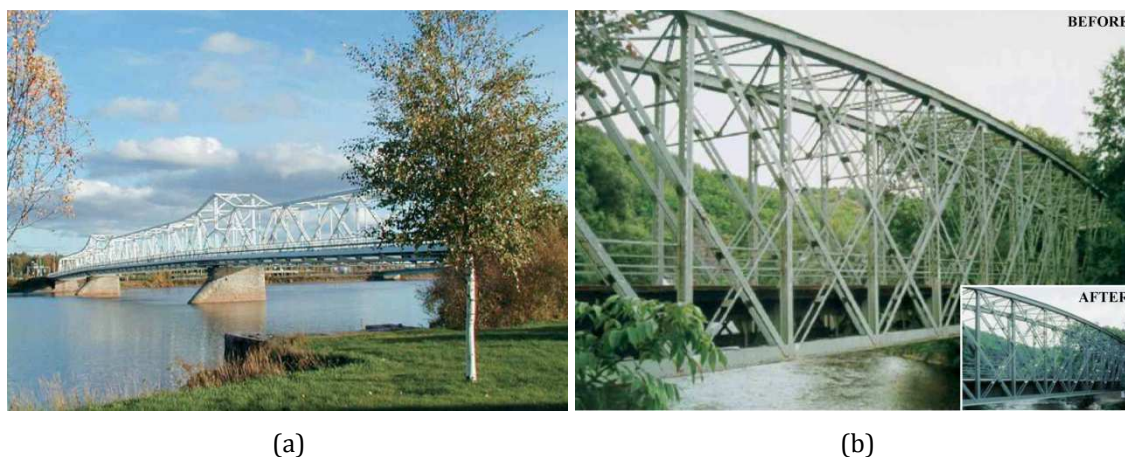
Figure 4.2 - Rehabilitation projects of steel bridges in Europe: (a) Tornionjoki steel Bridge (Kääriäinen and Pulkkinen, 2002); (b) side view of the old Kamp Bridge (Holzinger et al. , 2002).
