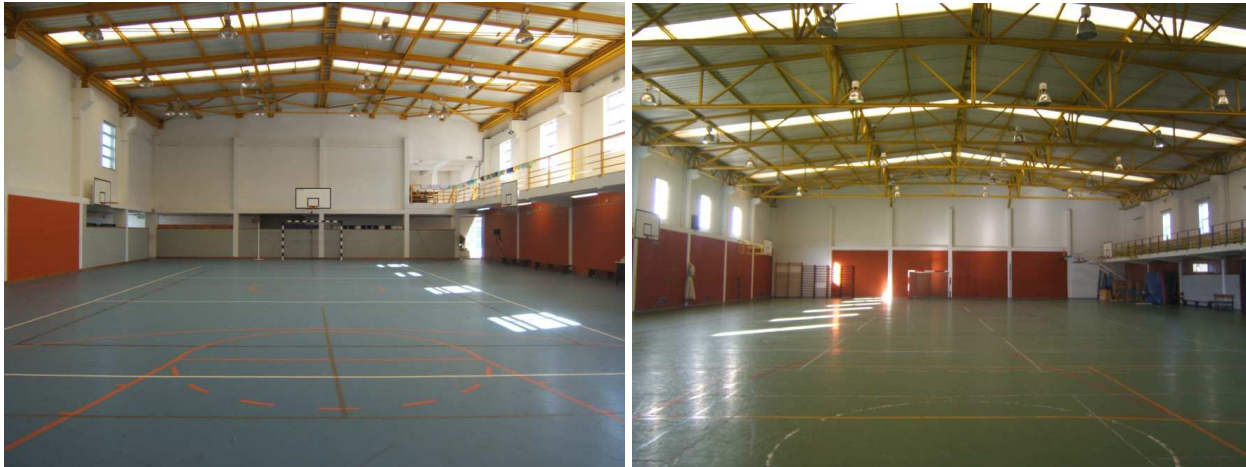
Figures 8 and 9 - Sports facilities n. 42 and n. 44.
