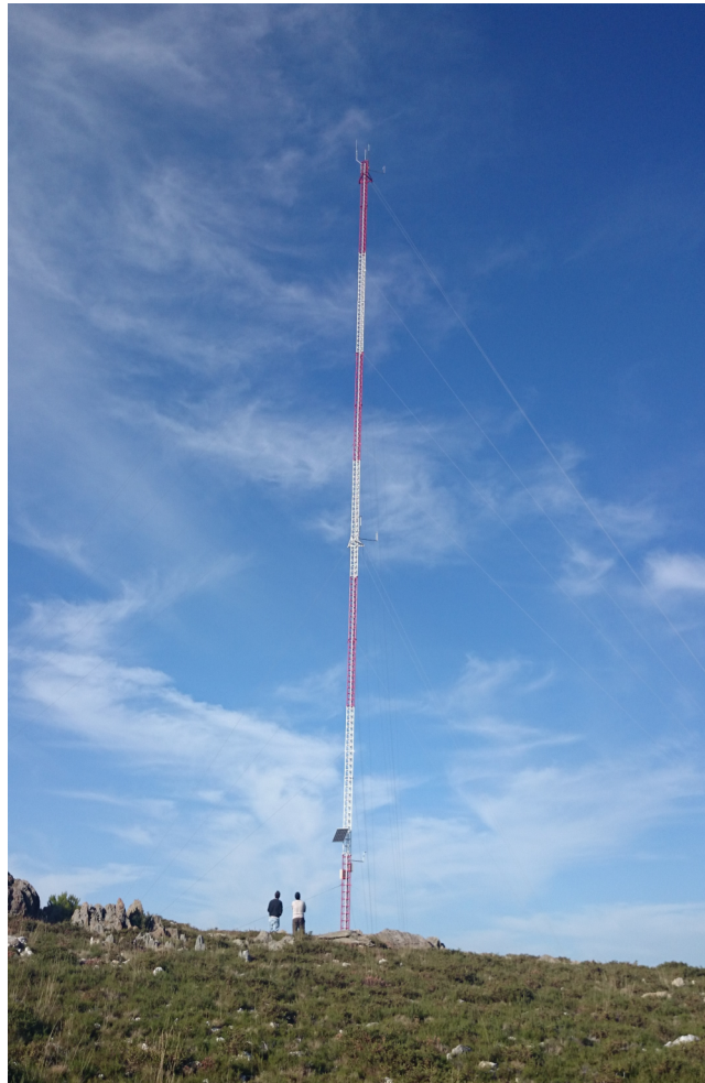
Figure 1.1: Measurement instruments mounted on a guyed triangular lattice mast located near Viseu, Portugal.
