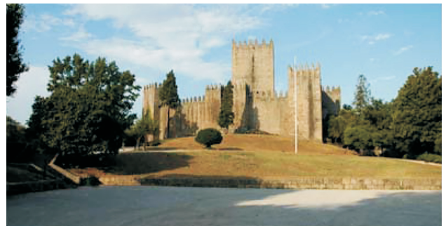
Figure 17 - A general view of the medieval Guimarães Castle.
