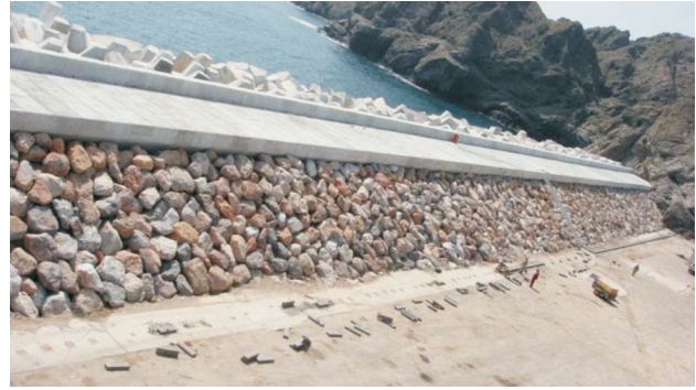
Figure 33 - View of the new protection of Jalali Fort.
