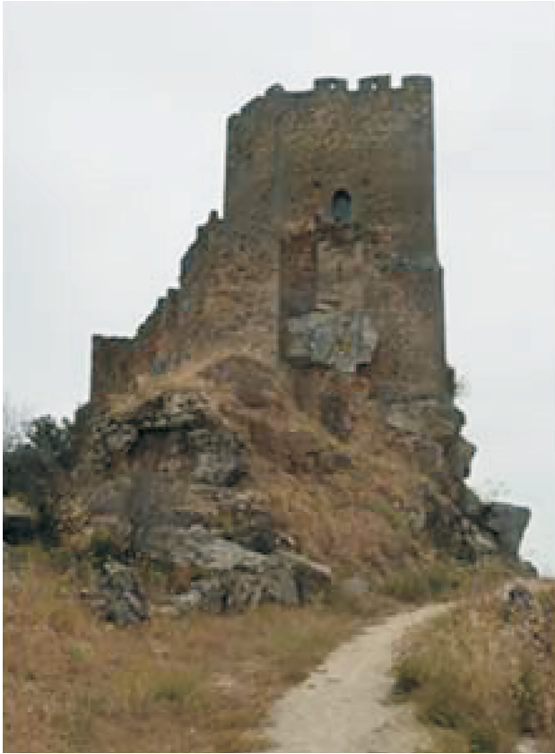
Figure 1 - Foundations of the medieval Algozo Fort.
