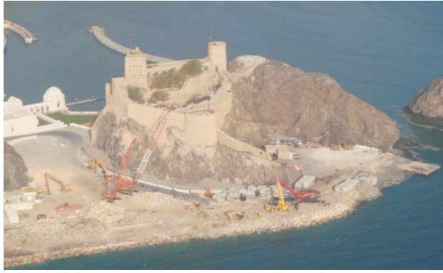
Figure 31 - Jalali Fort during construction of the seawall.
