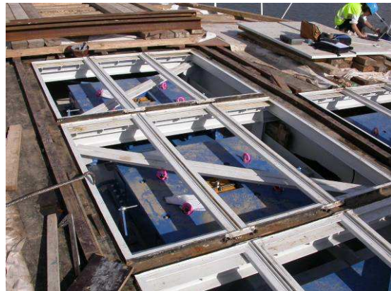
Figure 4: Horizontal TMD installed at the mid-span section
