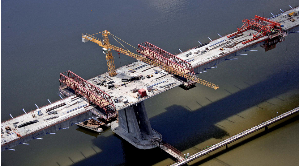
Figure 8.1 : Aerial view of Lezíria Bridge – May 2007 (© F. Piqueiro / Foto Engenho).
