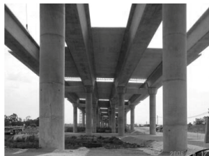
d) precast planks positioning.
