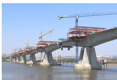
c) main bridge.
