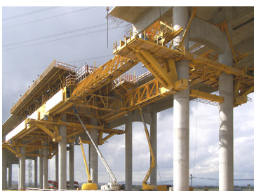
b) north approach viaduct.
