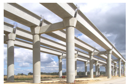
d) south approach viaduct.
