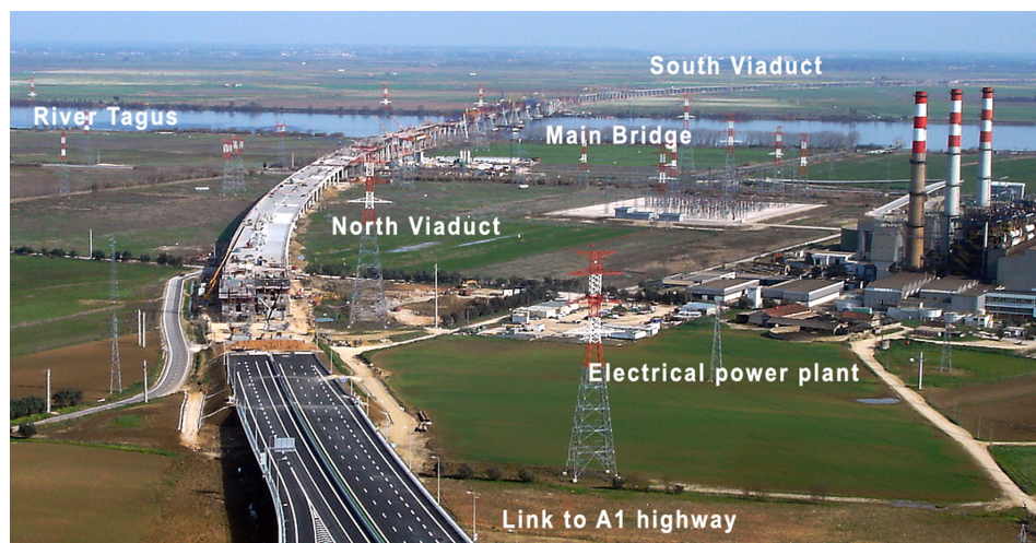
Figure 7.1 : Lezíria Bridge – construction stage at May 2007 (© TACE).
