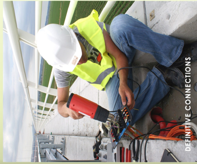
DEFINITIVE ACQUISITION NODES INSTALLATION
