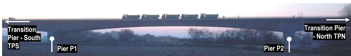
Figure 3.10 : Sorraia Bridge – Load test.
