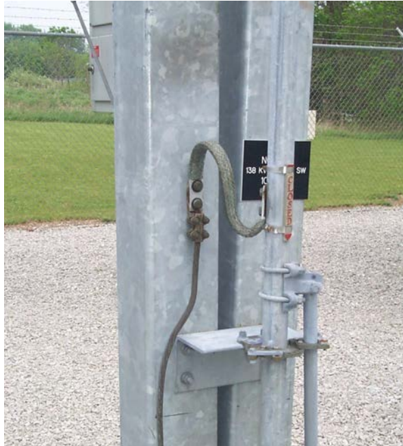
Figure 35—Typical braided ground
