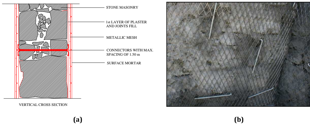
Figure 2.9. Reinforced connected plaster operation: a) schematic representation; b) application.
