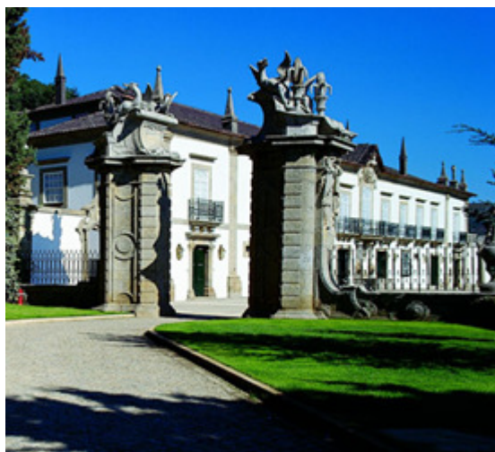
Fig. 3.29 – Solar da Rede, fachada principal [54]
