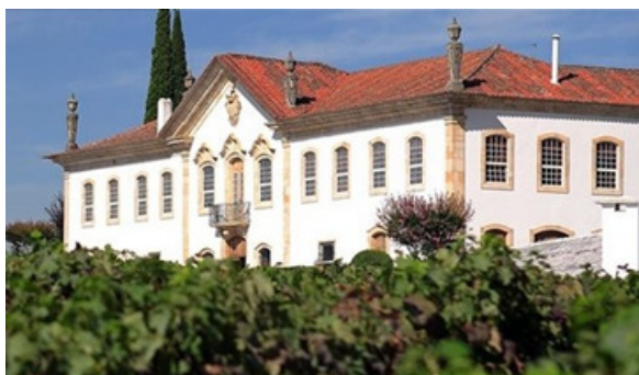
Fig. 3.4 – Quinta do Côtto, fachada principal [48]
