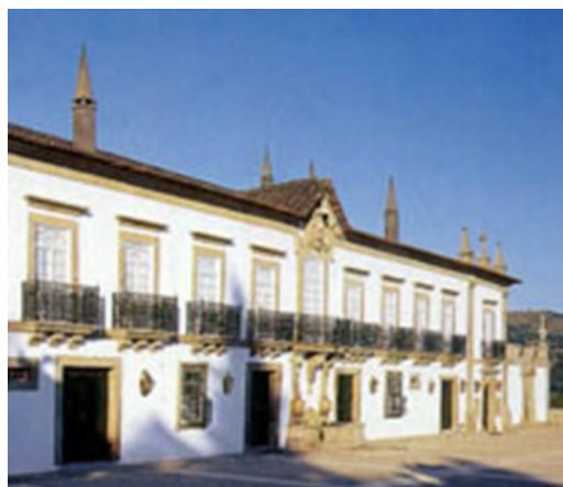
Fig. 5.2 – Solar da Rede, fachada principal [62]
