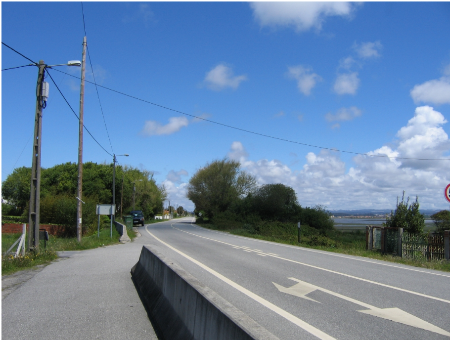
Figure D.2: N 327 - Facing North (Second Mobile Testbed)
