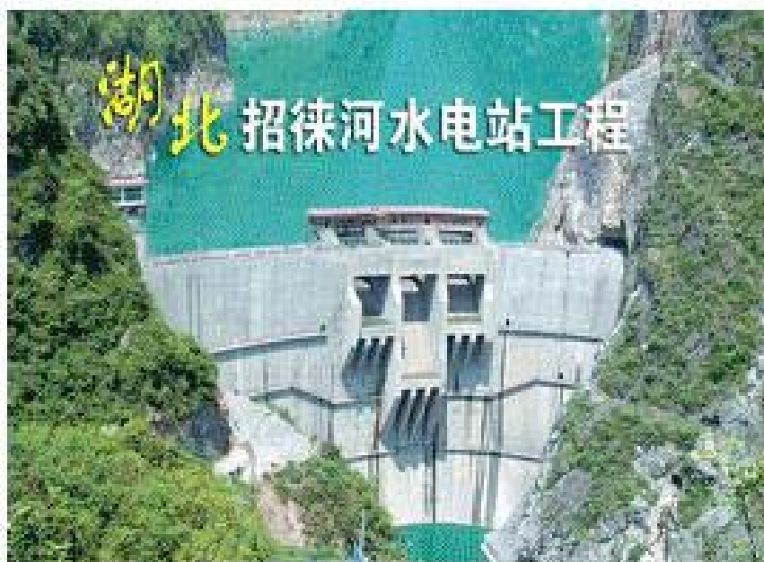
Figura 41 – Barragem de Zhaolaihe ( http://www.cwb11.com/jushudanwei/hasgj.html )
