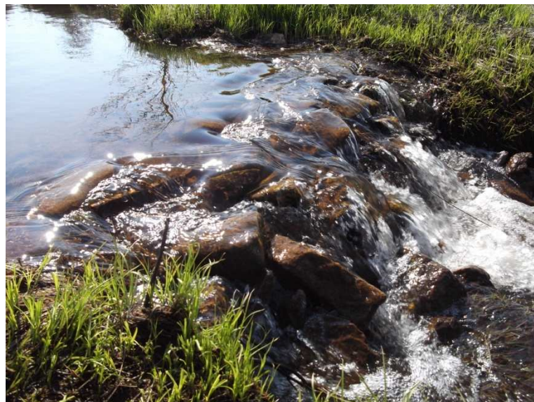
Fig.24 : Step built with rocks (by Jan Říha)
