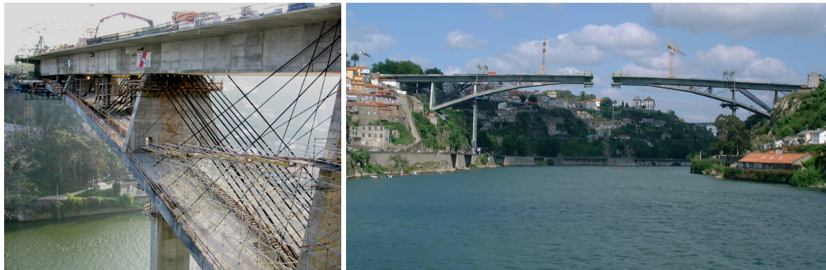
Figure 5.2 – Bridge during construction.
