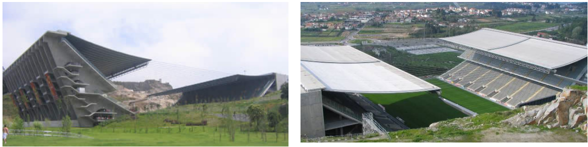
Figure 6.1 - Braga Municipal Sports Stadium (lateral view from the east side and top view of the roof from the west side).
