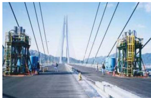
Figure 2.2 – Shakers used in the Forced Vibration Tests of Tataro cable-stayed Bridge in Japan
