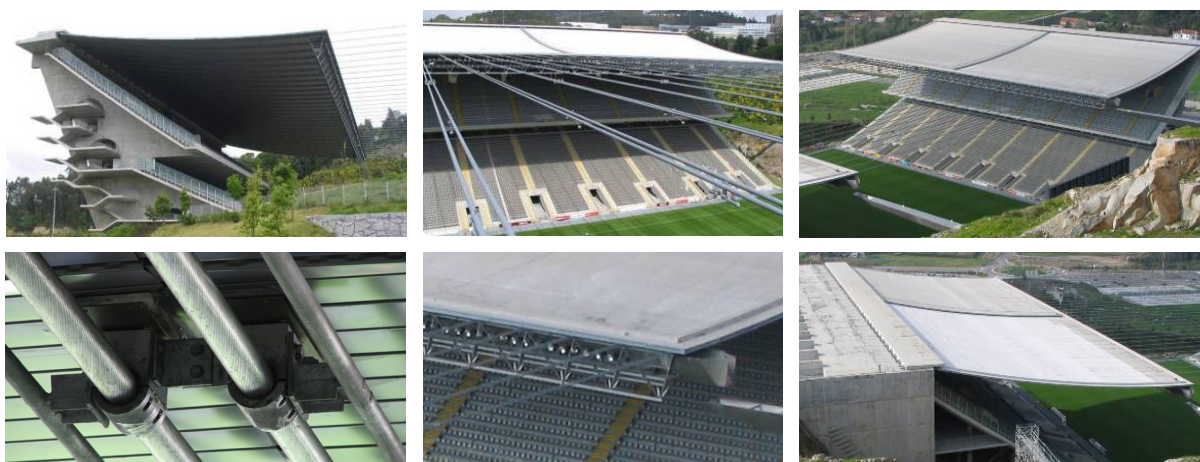
Figure 6.3 - Views of Braga Stadium (east stand, cables of the roof, slab of the east stand, detail of the connection between the cables and the slab, detail of the triangular truss in the inner border of the east slab and west slab).
