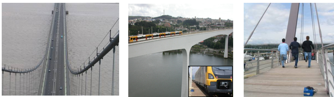
Figure 1.1 – Dynamic test of the Humber Bridge during normal operation, of the S. João Bridge (Porto, Portugal) during the passage of a train and of a cable-stayed footbridge (Viana do Castelo, Portugal) crossed by a group of three pedestrians.
