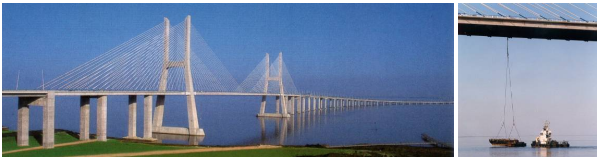
Figure 3.49 – Vasco da Gama Bridge (general view and barge suspended for application of the impulse)
