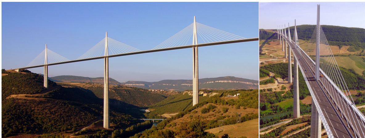
Figure 3.4 – Millau Viaduct over the valley of river Tarn; views of the tallest pier.
