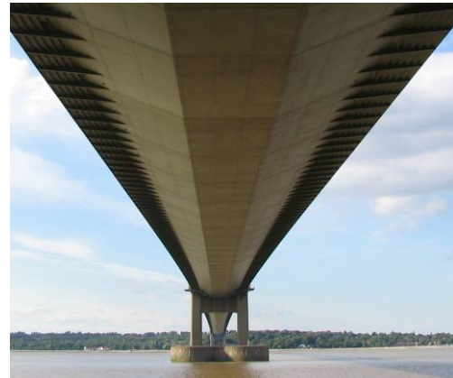
Figure 3.23 – Humber Bridge deck, view from underneath.
