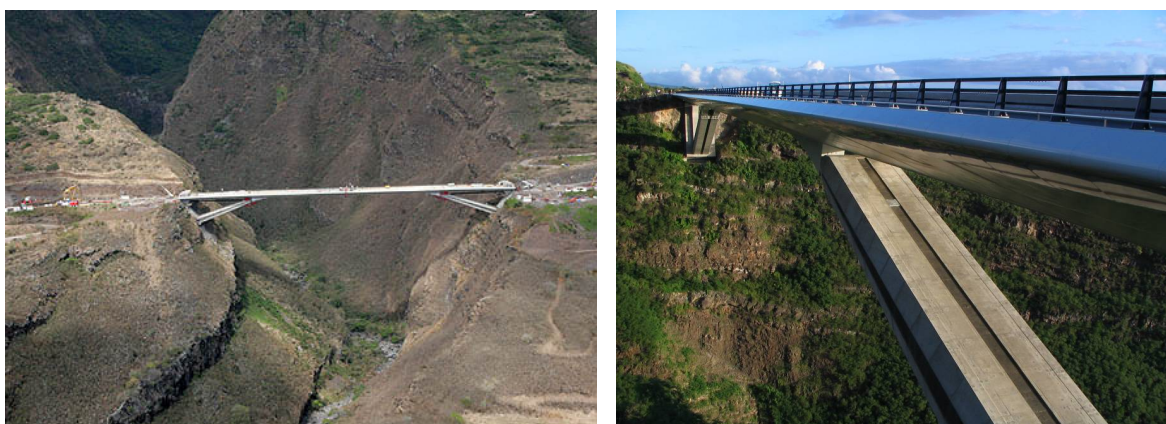
Figure 3.54 – La Grande Ravine Bridge, during construction (photo from www.greisch.com ) and after completion.
