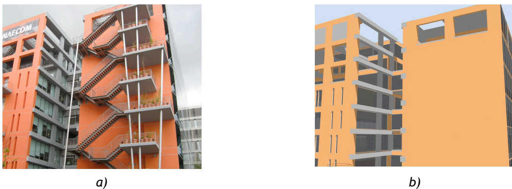
Figure 41 - Images of a) the existent building and b) the model used on EP
