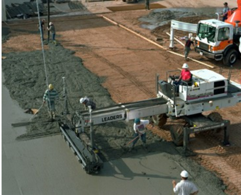
Fig.3.8 – Utilização do Laser Screed ( http://www.concreteenterprises.com/Photo%20Gallery.htm ).
