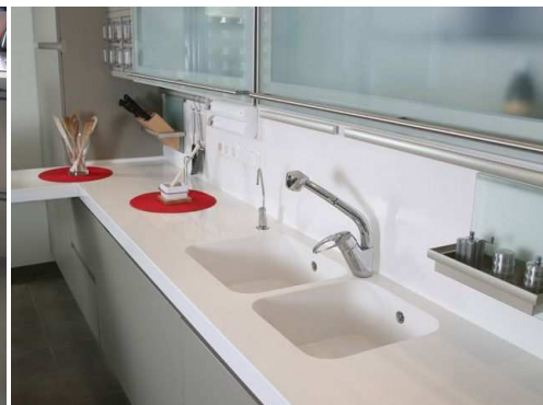
Fig.3.29 – Tampo de silestone
