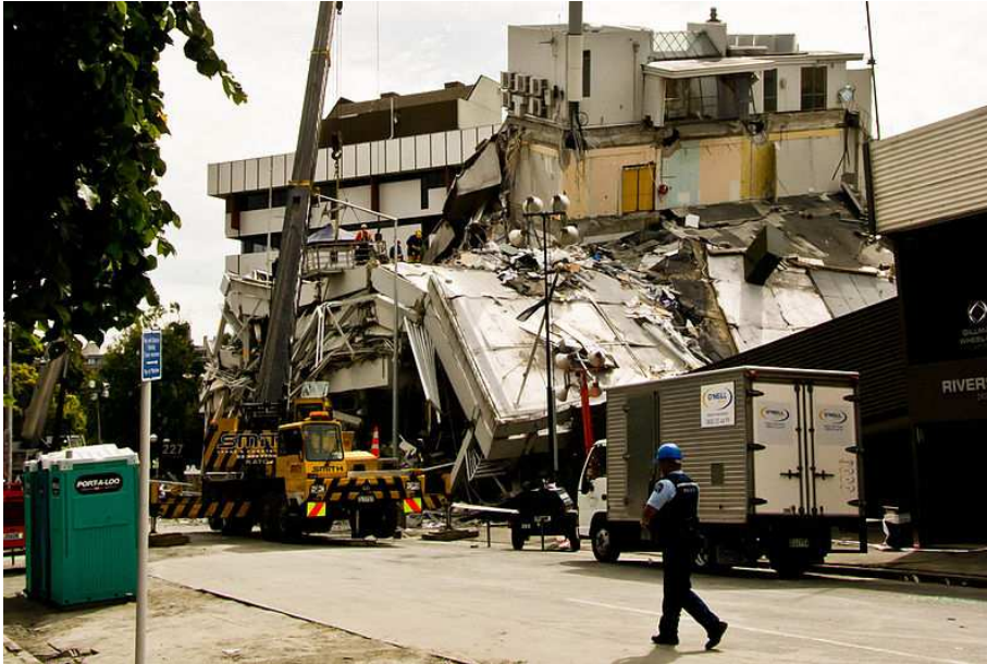
Figure 2.12 – The Pyne Gould Corporation (PGC) Building following the 2011 Christchurch earthquake.
