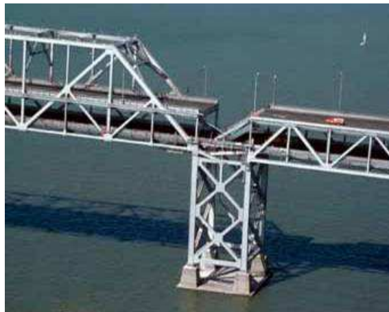
Figure 2.3 – Oakland Bay Bridge: collapsed portion of the upper deck.
