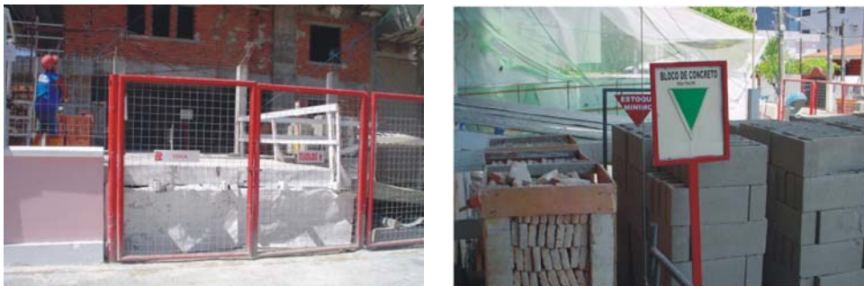
Figure 15 – Unloading dock (left) and signalled storage area (right) at a construction site in Fortaleza. Source: Miranda Filho (2008)
