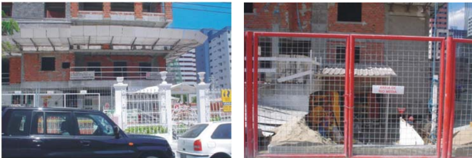
Figure 13 – Transparent fence (left) and gate (right) surrounding a construction site in Fortaleza. Source: Miranda Filho (2008)
