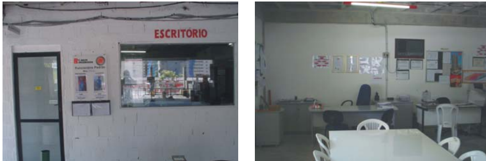
Figure 16 – Site office with glass windows and doors (left) and with no internal divisions (right) at a construction site in Fortaleza. Source: Miranda Filho (2008)
