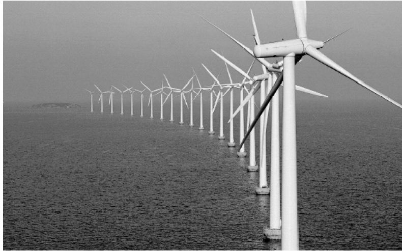
Figure 3.5 - Carbon fibres will be employed in wind turbine blades over 50m long. Source: Reinforced Plastics.
