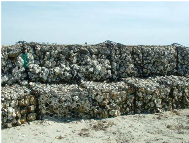
Fig.2.9 – Esporão formado por gabions ( http://www.conservancy.co.uk/learn/wildlife/process.htm ).
