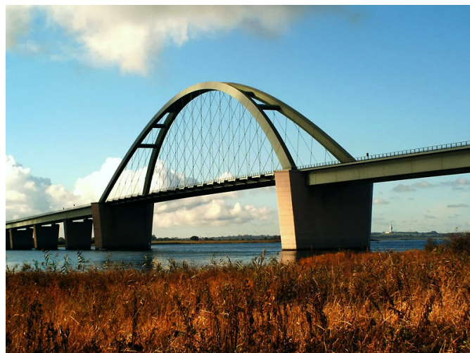
Fig. 3.13 – Fehmarnsund Bridge – Germany [22]
