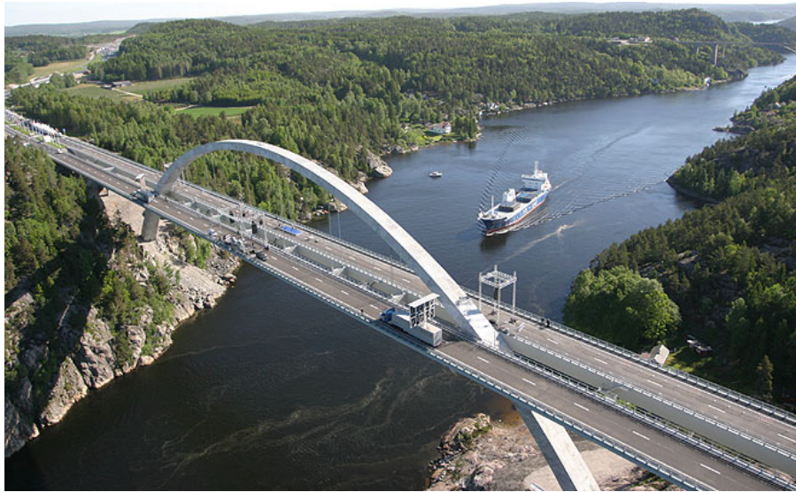
Fig. 2.6 – Svinesund Bridge – Norway/Sweden border [9]
