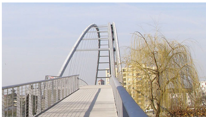
Fig. 2.13 – Tri-Countries Bridge - Weil am Rhein – France/Germany [16]
