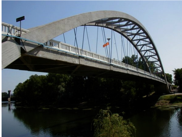
Fig. 2.12 – Castelmoron Bridge - Castelmoron-sur-Lot [15]
