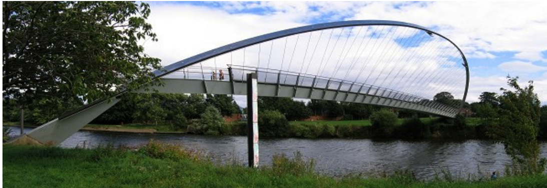
Fig. 2.8 – York Millennium footbridge – York [11]
