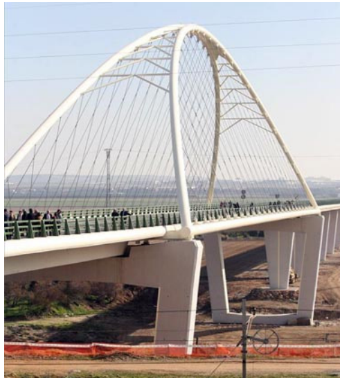
Fig. 3.14 – Palma del Rio Bridge – Spain [23]
