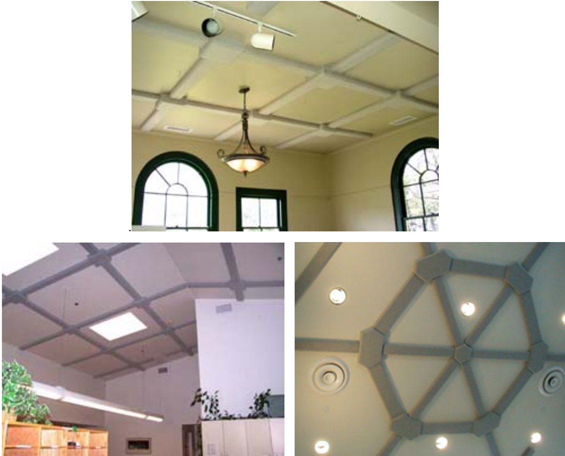
Fig.5-4 (A, B e C) – Coffered ceiling system da ASC [37]
