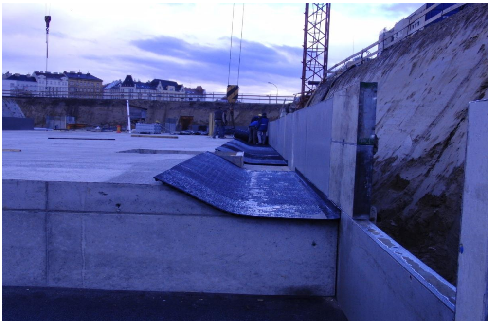
Figure 4.1 – Elastic foundation of the building
