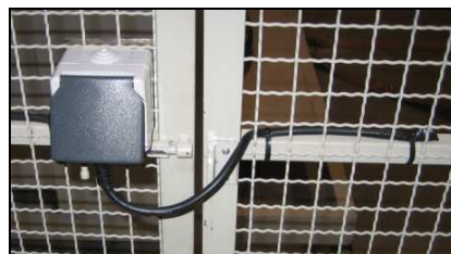
Figure 8.3 - Example of a limit switch (OMRON Industrial Automation) on the left, and the safety system of the Faraday cage on the right.
