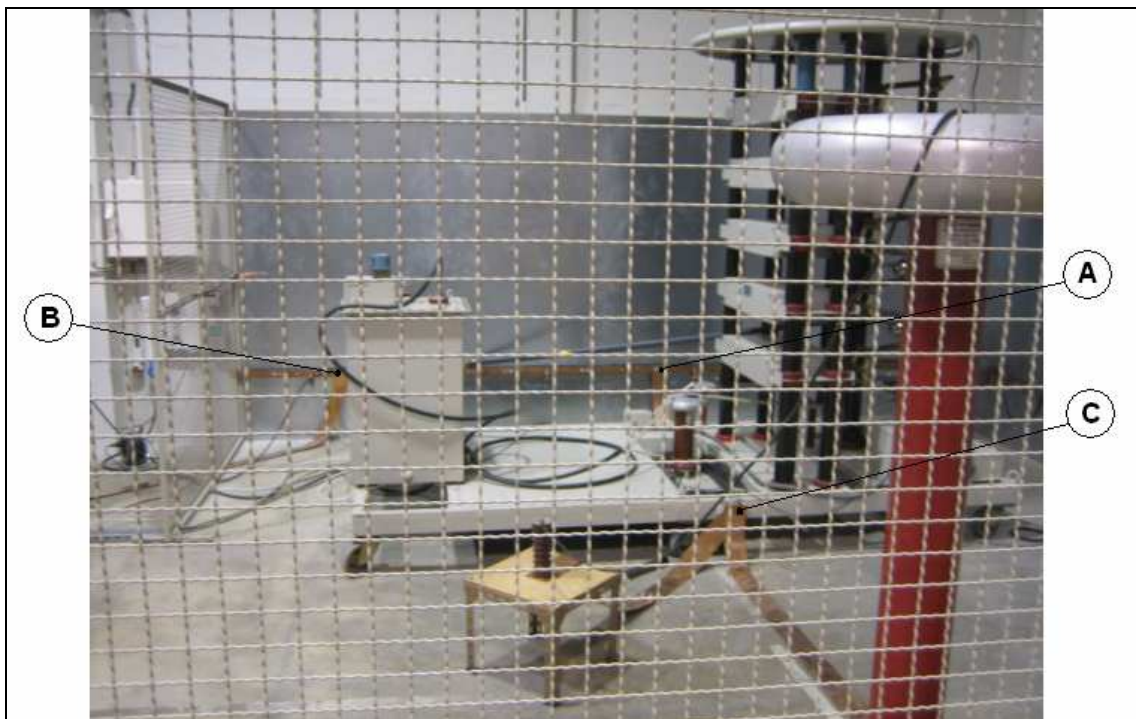
Figure 3.19 - Detail of the earth connections of the equipment: points (A), (B) and (C).
