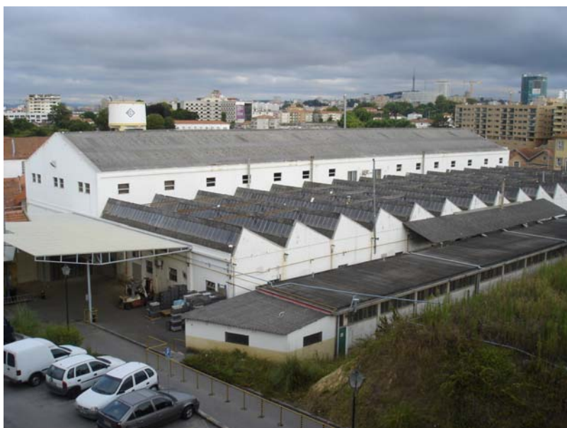
Figura 1 – GE Power Controls Portugal
