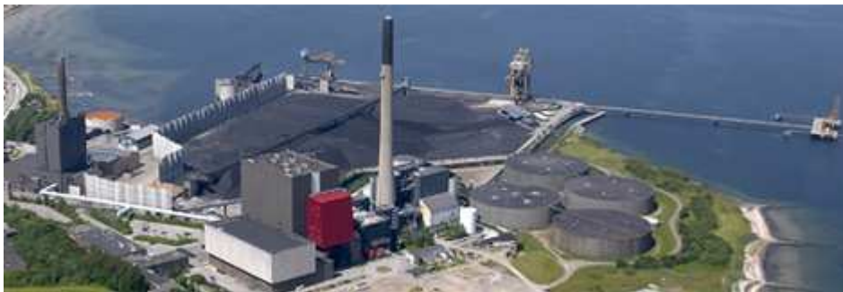
Figure 2.26 - Ensted Power Station. Source : Dong Energy
