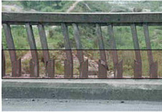
Figura 2.8 – Pilares colapsados na ponte de Hsiaoyudong (Lin *et al.* (2008))
