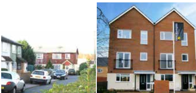
Figure 1 Typical owner occupied properties in Stanwell before and after the scheme
