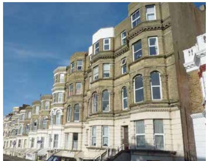
Figure 2 - Georgian terrace in the Renewal Area
