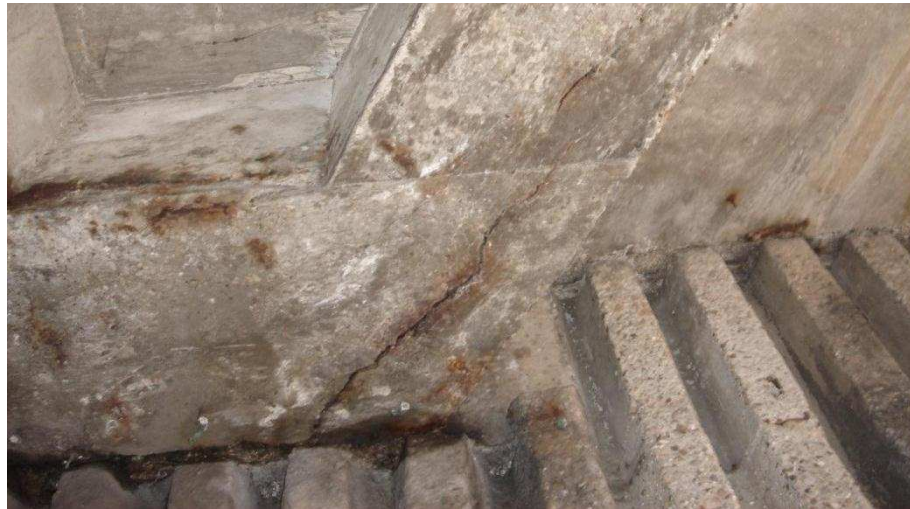
(a) Visual Inspection on 06/07/2010
