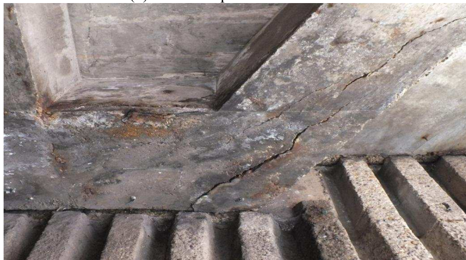
(c) Visual Inspection on 29/07/2012
