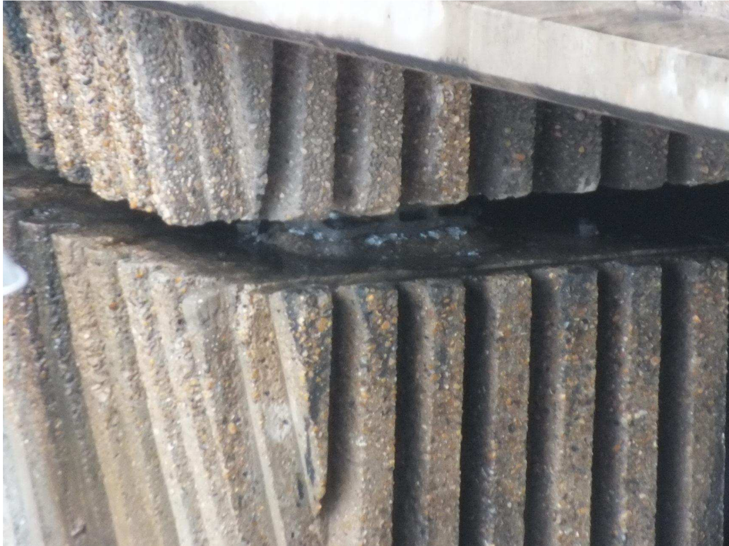
Figure D.5 – Pier 2 Bearing
