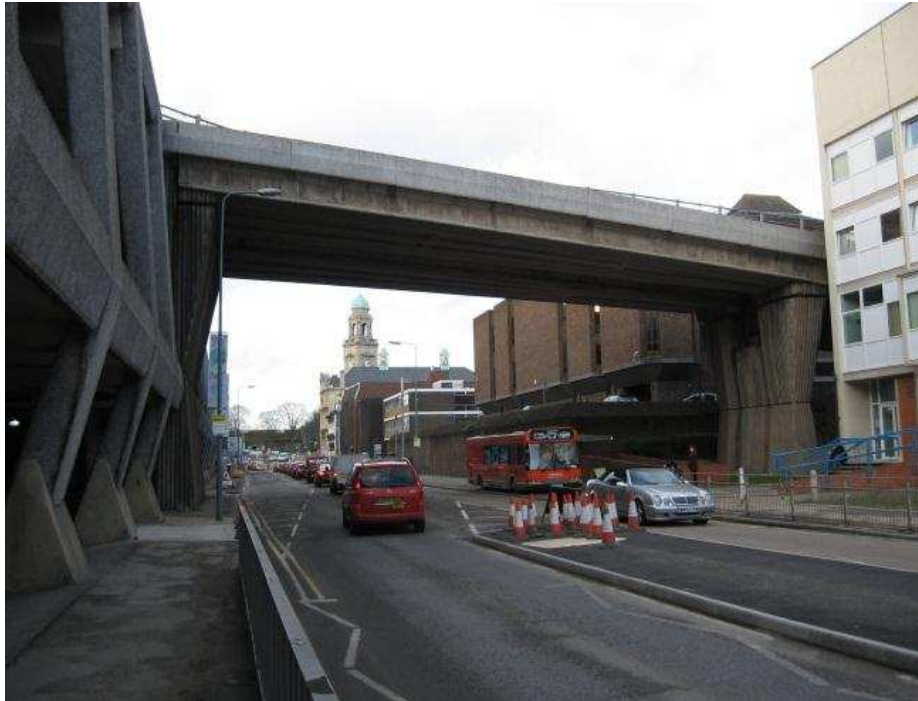
Figure D.15 – South view of Span 1
