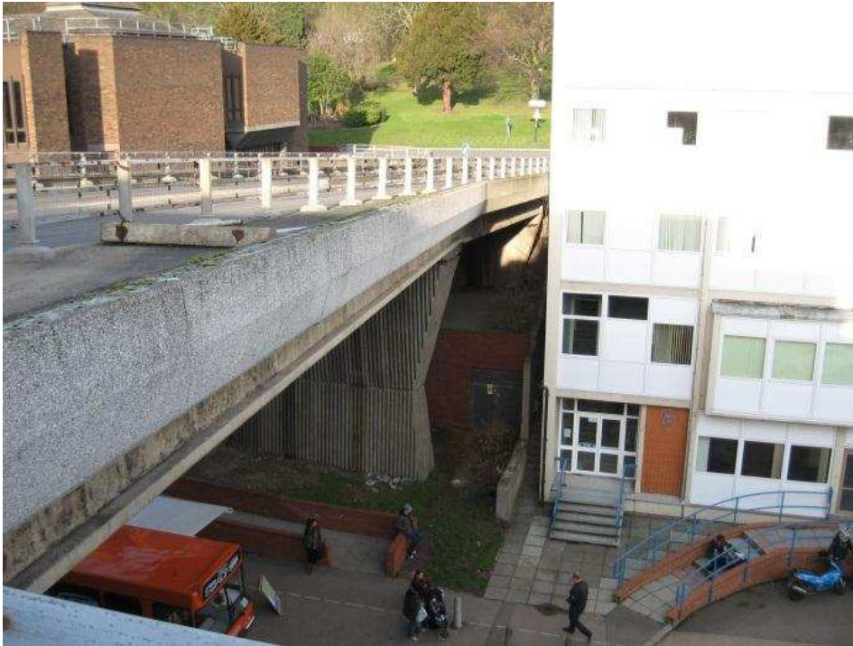
Figure D.19 – South Edge Beam and Parapet
