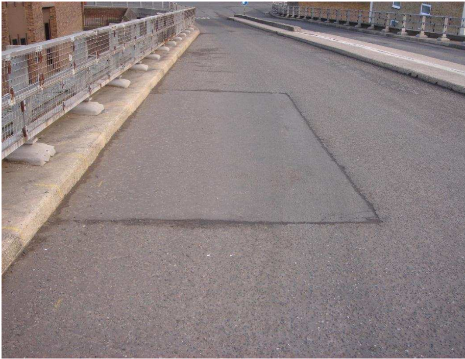
Figure D.21 – Span 1 reinstatement view
