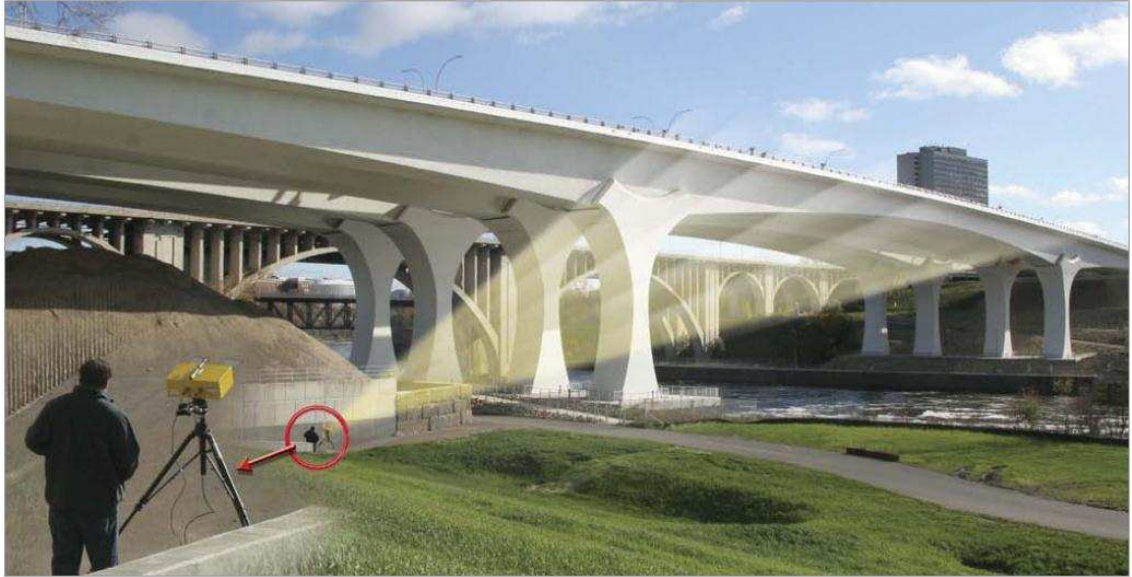
Figure 2.22 – Dynamic monitoring of a full-scale bridge with IBIS-S (Ids ltd., 2012)
