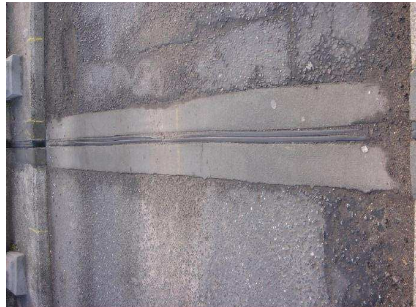
Figure D.14 – Expansion joints between span 3 and 4
