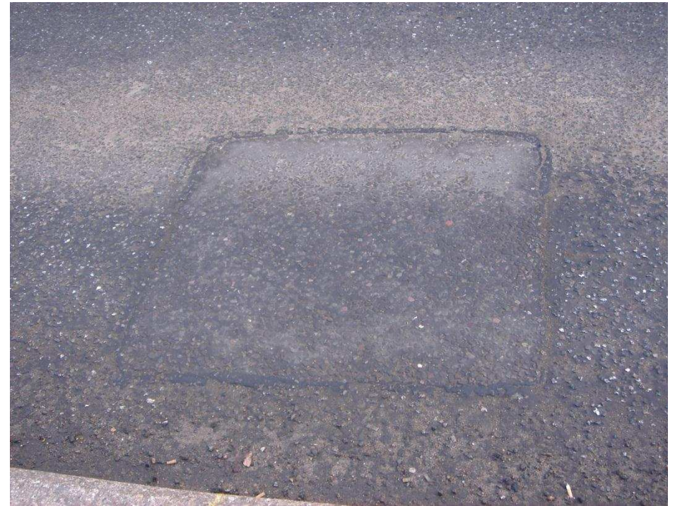
Figure D.22 – Span 4 reinstatement view
