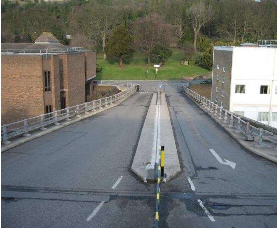
Figure D.17 – West View of structure
