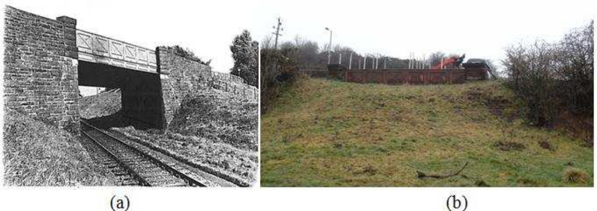
Figure 4.15 – Historic and recent view of the Darvel Road Bridge. (Wikipedia and Picture by Gokhan Kilic, 2010)
