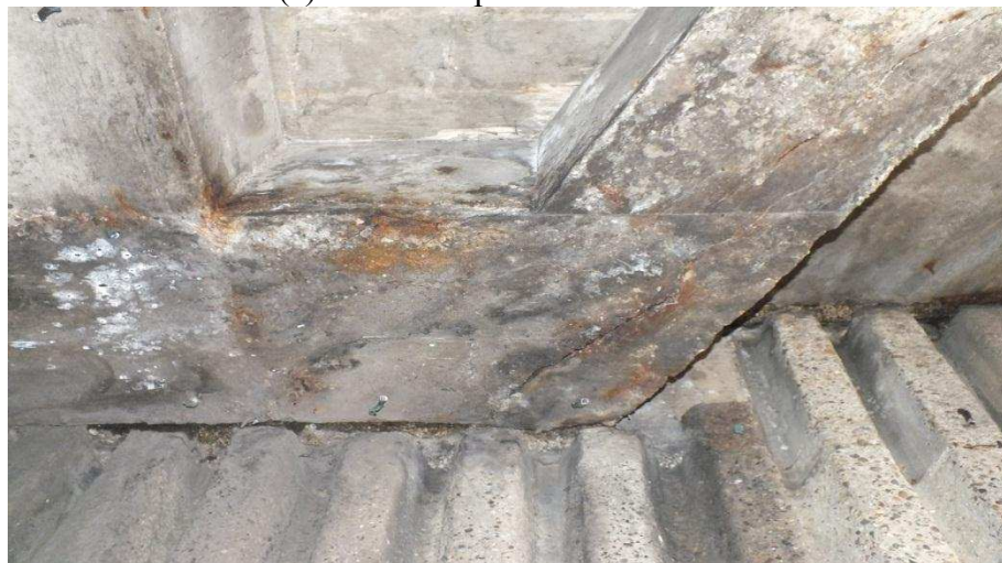
(b) Visual Inspection on 25/06/2011
