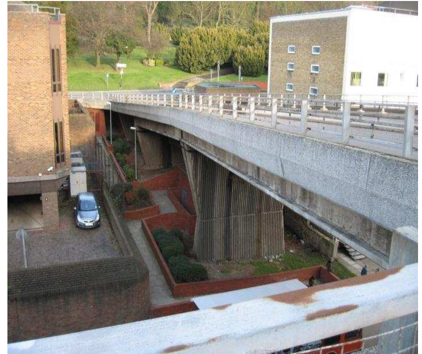
Figure D.20 – North Edge Beam and Parapet
