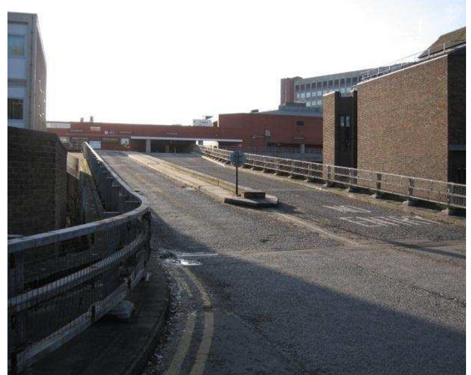
Figure D.18 – East view of structure
