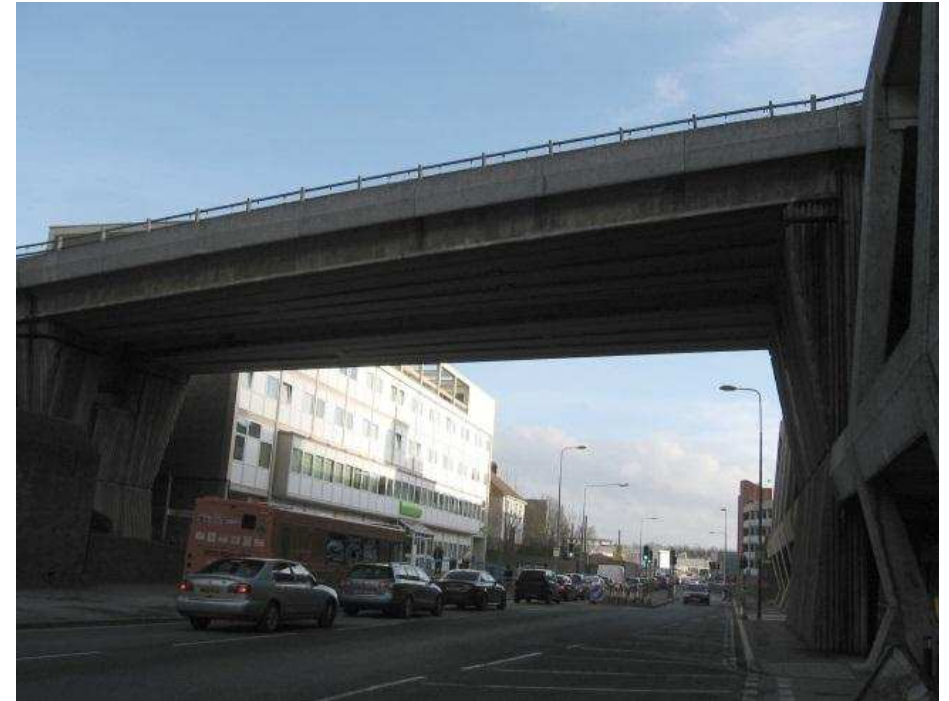
Figure D.16 – North view of Span 1
