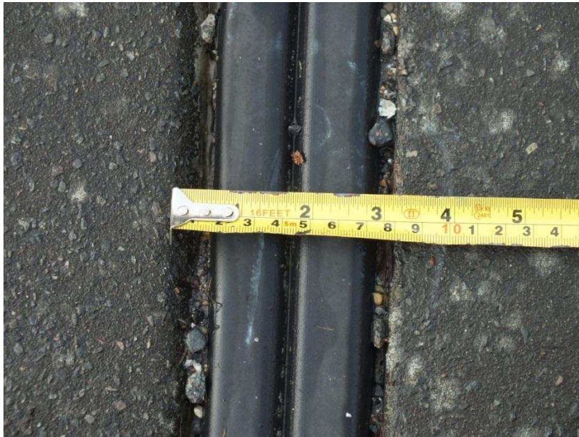
Figure D.13 – Expansion span 1 and 2
