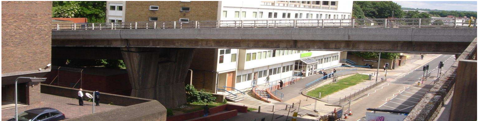
Figure D.1 - General view of the Pentagon Road Bridge (North Elevation)
