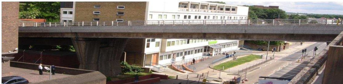
Figure 4.28 – View of Pentagon Road Bridge (Photos from Gokhan Kilic, 2010)
