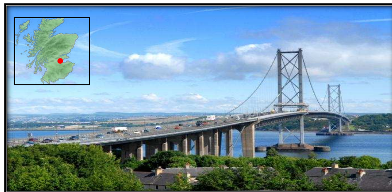
Figure 4.4 – General view of the Forth Road Bridge (Forth Estuary Transport Authority, 2010)
