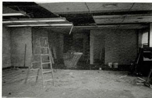
The Learning Resource Center during construction...
