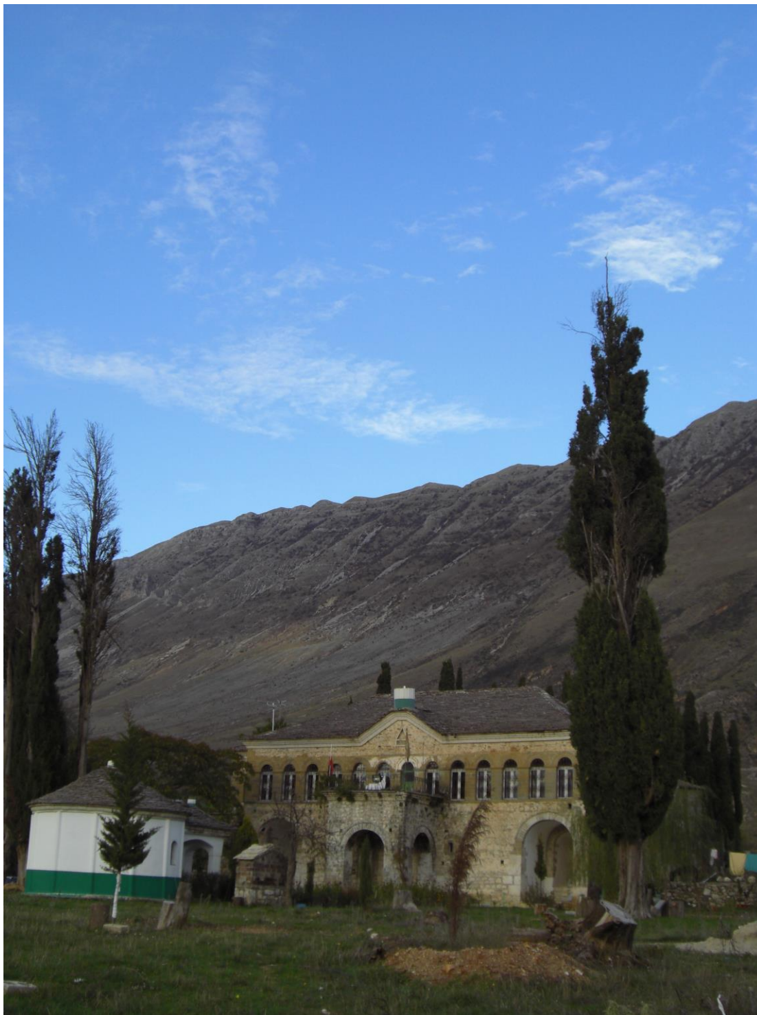
Figure 3.2. The Melan Tekke and newly repaired shrine. Gjirokastrë, 2007.
