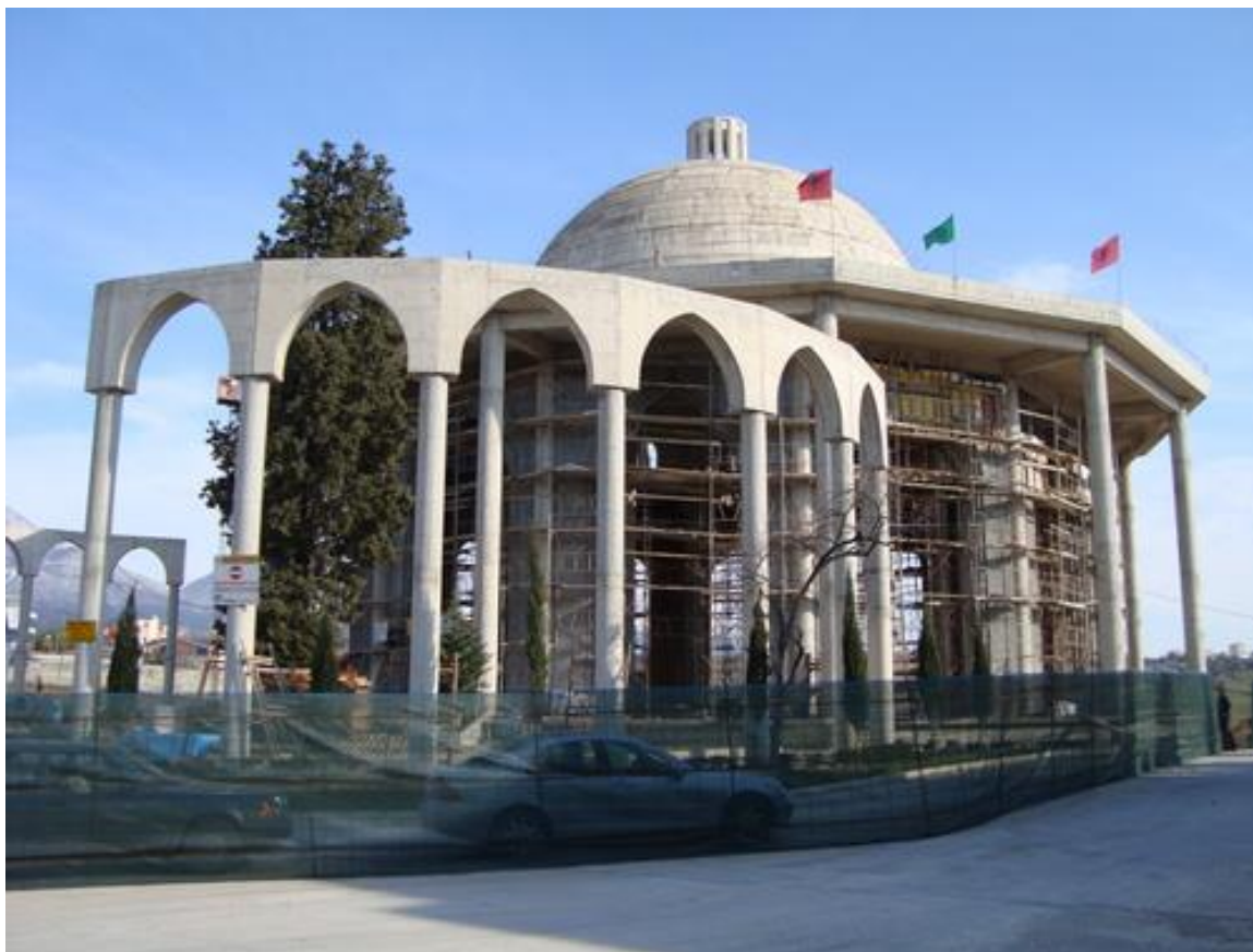
Figure 3.5. The prayer house under construction. Tirana, 2007.
