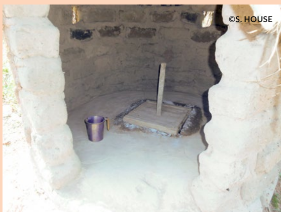
A very old woman who is also blind can squat but she finds it difficult to hit a standard sized hole. This hole has therefore been made larger by her son who built the latrine for her. ( Nigeria )
