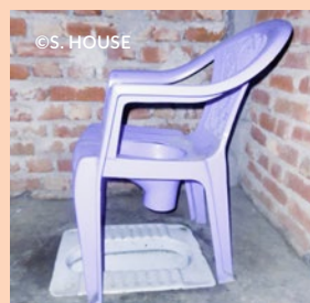
Plastic pre-formed toilet chair with a chute brought in the local market ( Nepal )
