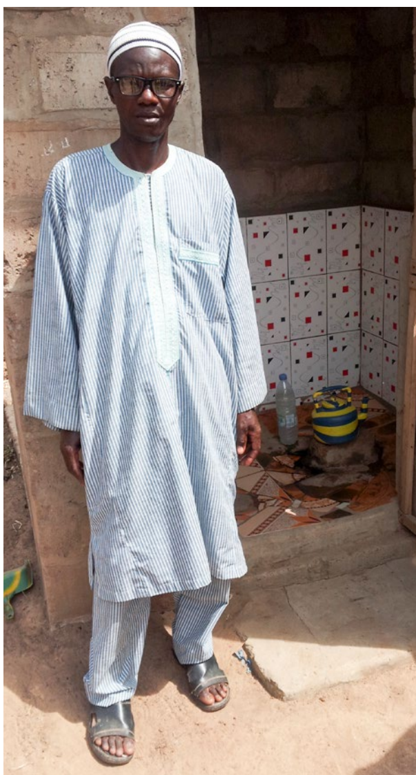
UPGRADED TOILET PARTIALLY CONSTRUCTED WITH EXTERNAL DONOR FUNDS, FOLLOWING ODF DECLARATION. ©SUZANNE FERRON
