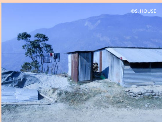
A temporary household latrine in Rasuwa, Nepal , shared by two families after the devastating earthquake. Next to the latrine is a child's potty.
