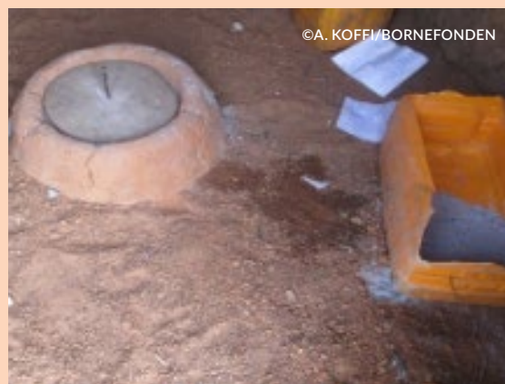
Slightly raised latrine hole that can be sat on or squatted over, constructed for N'ingmayo who is visually impaired. It helps her position herself over the drophole ( Togo )
