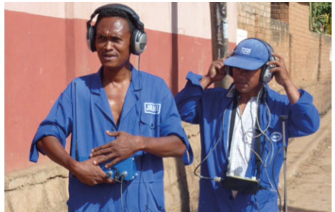
Image: JIRAMA NRW team conducting leak detection and repair. Credit: WSUP
