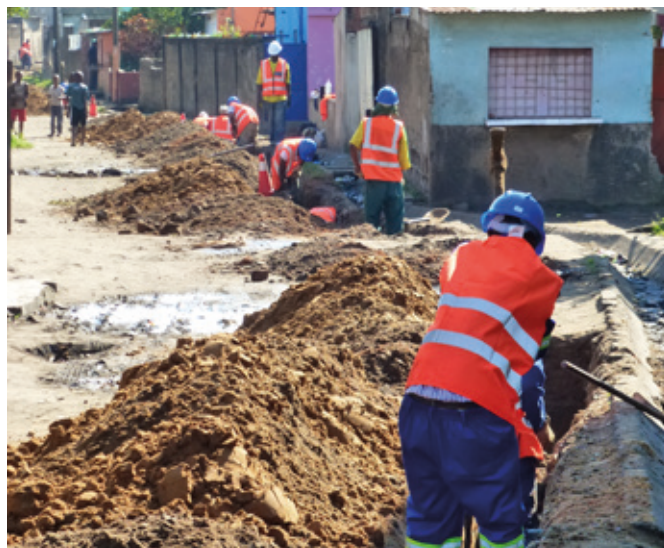
Image: Tertiary network construction in Chamanculo, Maputo. Credit: WSUP
