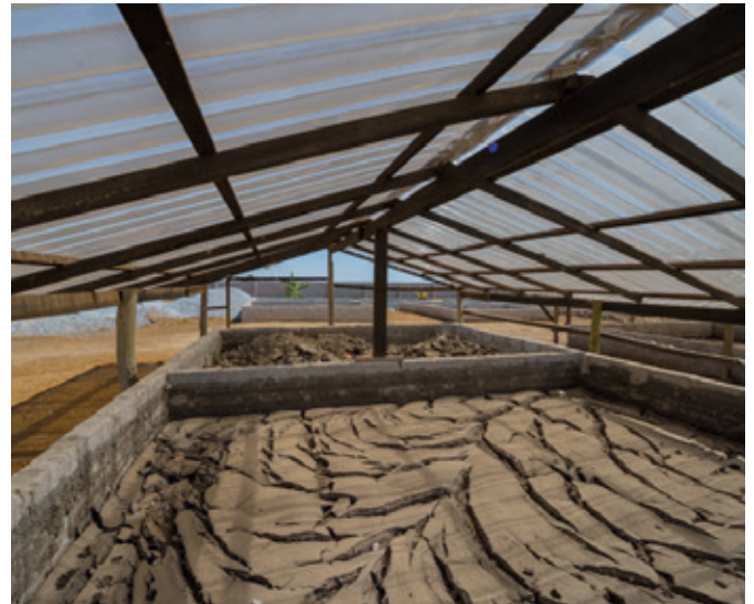
Image: Drying beds for treatment of sludge collected by the FSM service, Lusaka. Credit: Gareth Bentley.
