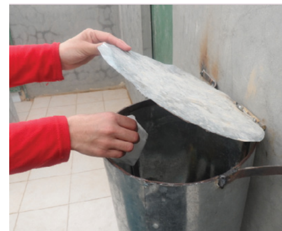
Figure 4 and 5: Direct disposal to a storage bin from a chute inside the cubicle (Oxfam-Nepal, 2015)
