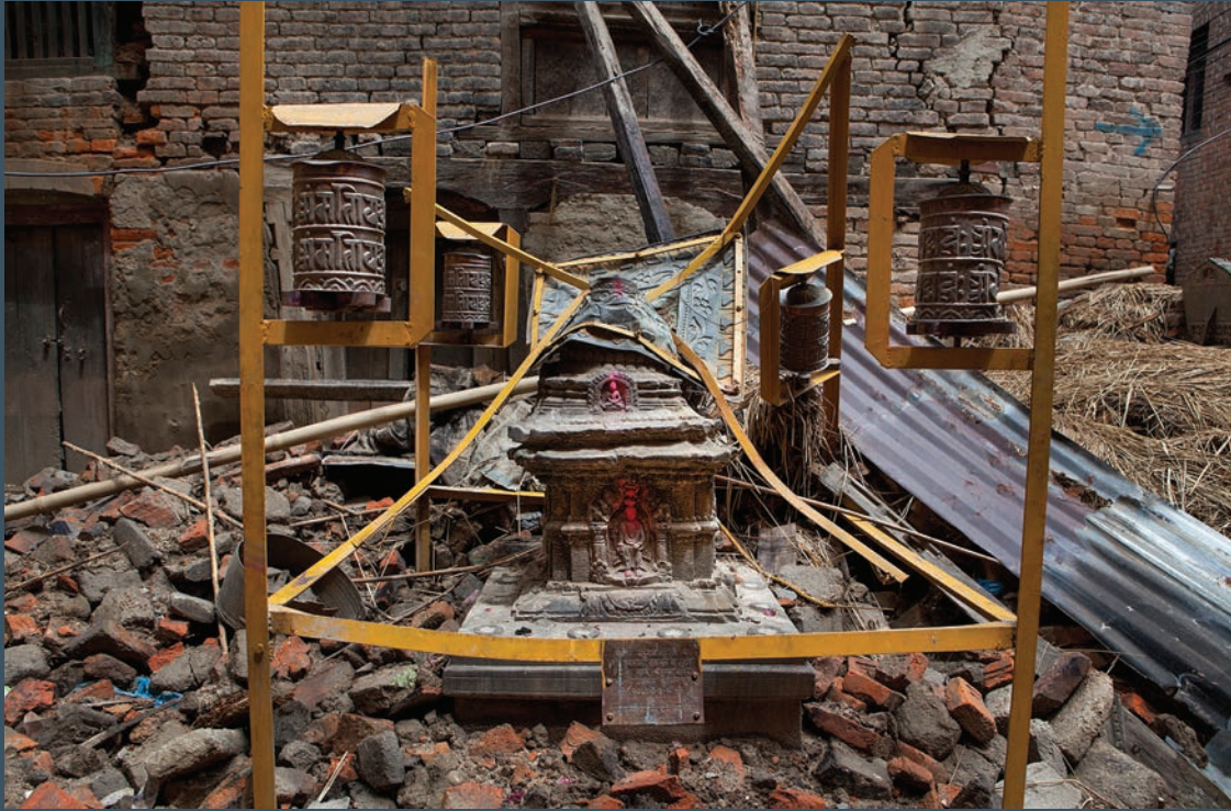
In the Chyusal neighborhood of Patan, Buddhist stone shrines, called caitya , and prayer wheels were damaged by falling brick and debris from the surrounding houses. This section of old Patan was damaged more severely than other neighborhoods.
