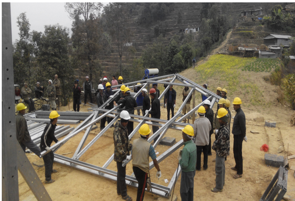
Figure 1. Villagers erect steel house frames under professional supervision.
