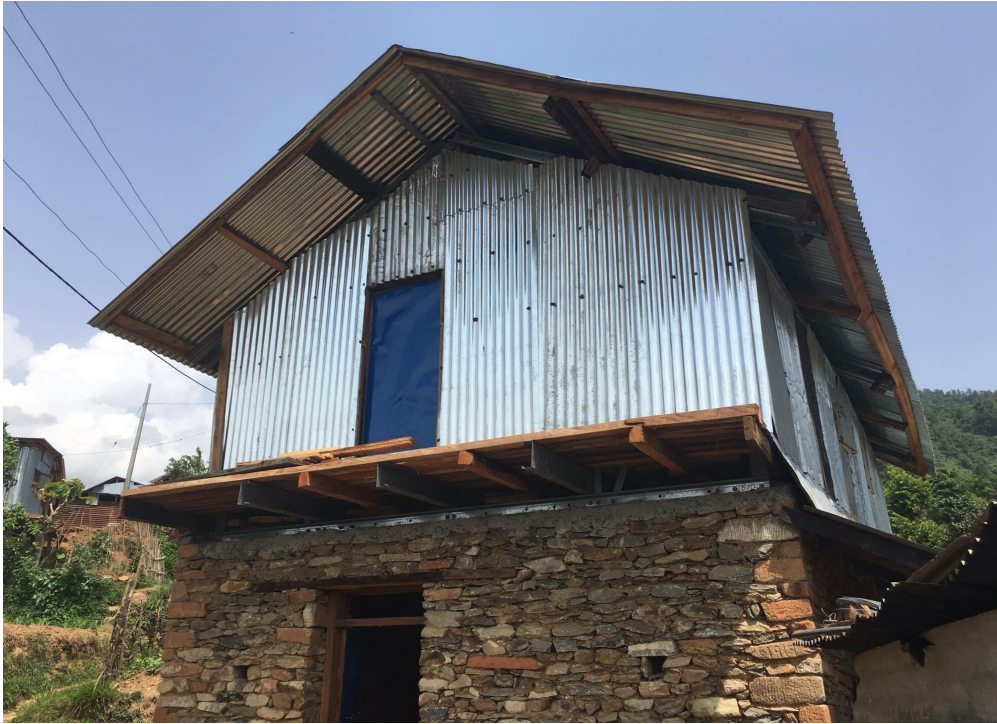
Figure 2. Rebuilt earthquake-resistant two-story local house.
