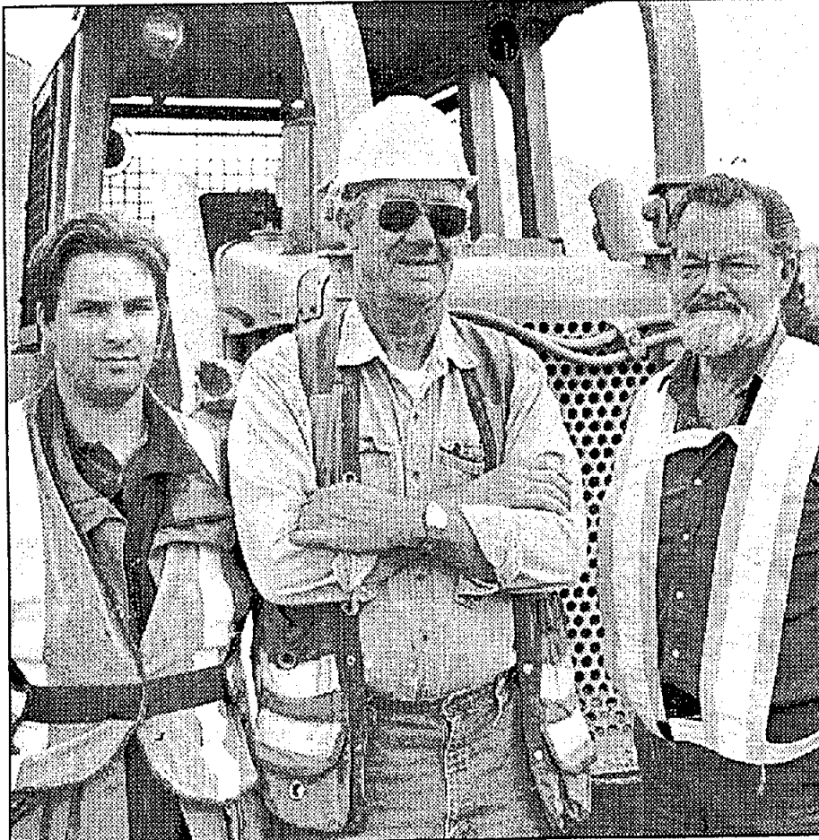
Along Hwy16, Dave Wolfe, Fran Grelson and Jim Mantel are working hard constructing the city's new linear park: the Grand Trunk Pathway. The park will bypass grounds contaminated by a now-defunct Federated Co-op bulk fuel plant.
