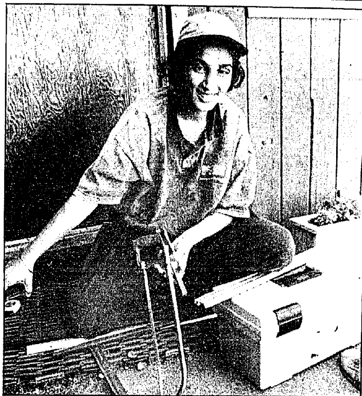
WEATHER STRIPPING on doors stops draughts and saves money. That's Kamaljit Buttar cutting a piece of weatherstripping to fit. She's one of two people in the area installing basic energy packages on homes. Nearly 1,000 homes here and in Kitimat will benefit by the BC 21 Power Smart program by this fall.
