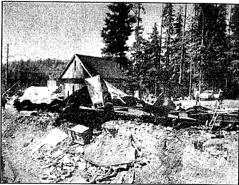
DONATIONS ARE being sought for Mike and Carol Horsburgh who lost their Nass Valley home to fire last week. The blaze destroyed all of their possessions but they were able to save their A-Z General Store building on the left.
