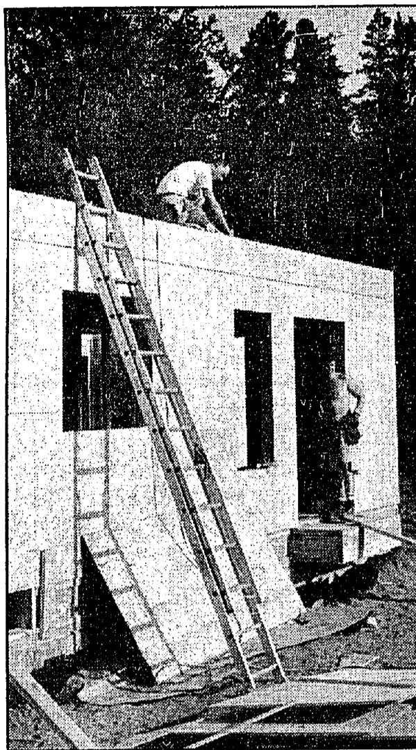
BUILDERS FROM MGB Developments work on a home in a new subdivision in the Mountain Vista area. Like other builders, they will have to wait several more months to find out exactly how new building regulations will affect their business.
