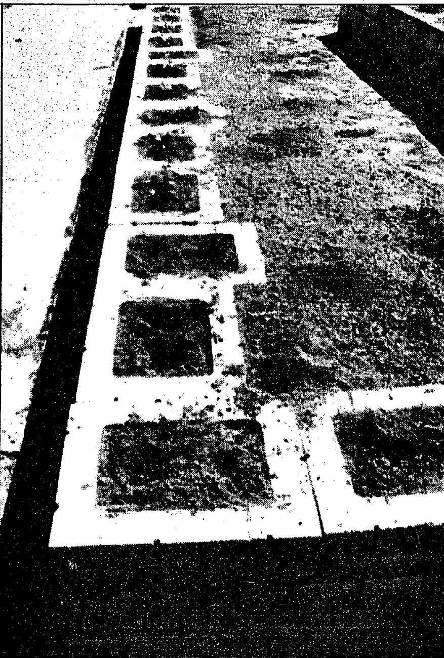
Construction on the new B.C. Access Centre went smoothly, but the landscaping hit a snag last weekend. Mary DaSilva put out bedding plants Friday to dress up the masonry wall bordering the parking lot, but discovered Saturday morning that about half the petunias and other flowers had been stolen overnight. "I wonder about the mentality of some people in this community", she remarked.
