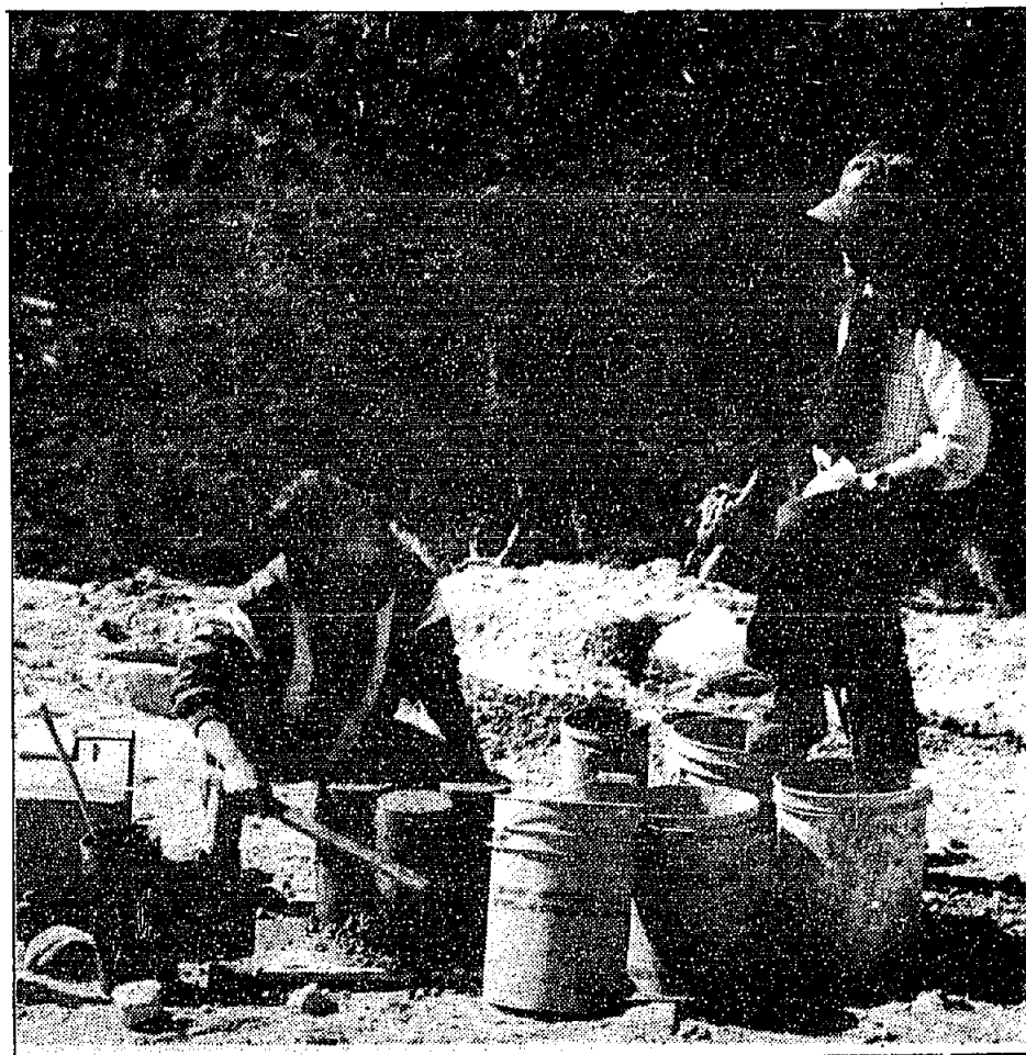
KARL ERNST OF MUELLER LIFTS oversees the testing of the concrete for the tower foundations on Shames Mountain. Lapoint Engineering conducted all the testing required by the Ministry of Highways, Aerial Tramways division.
