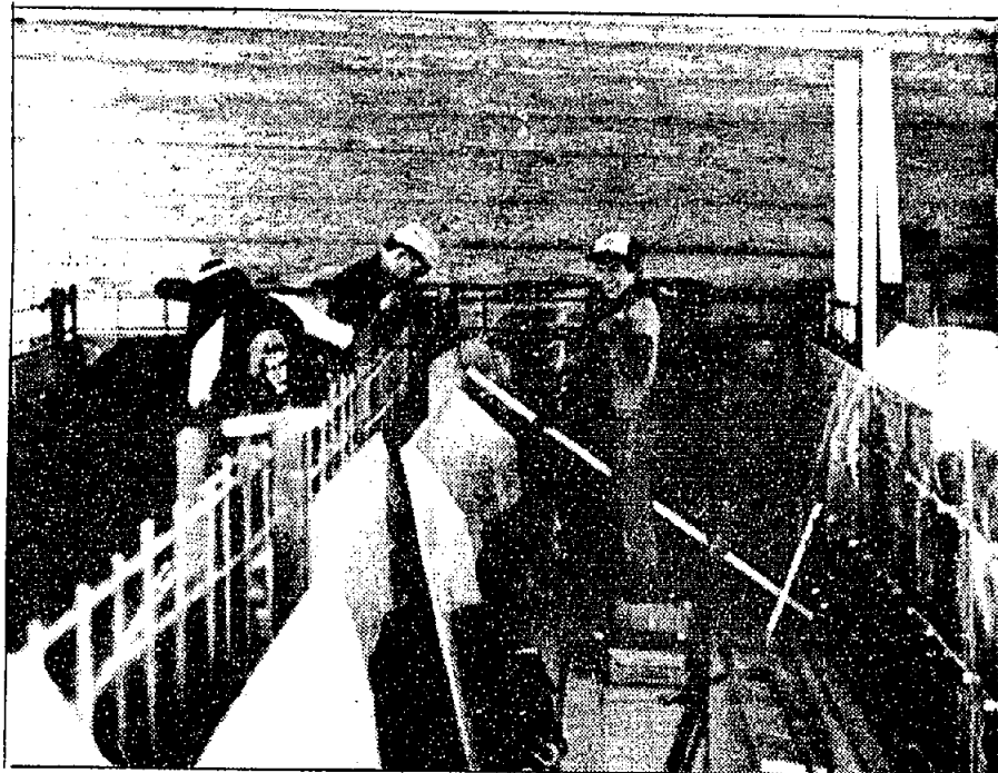
The new raceway at the Pine Lake Hatchery is nearing completion. When in operation, the raceway will hold an estimated 500,000 salmon fry, compared to 50,000 in a Capilano trough, significantly increasing the output of the hatchery. Here, Ministry of Fisheries engineer/technician, Norm Hill, inspects the facility while Challenge '87 students, Rod Bolan and Lyle Bolton, clean the raceway in preparation for pouring the concrete center divider.
