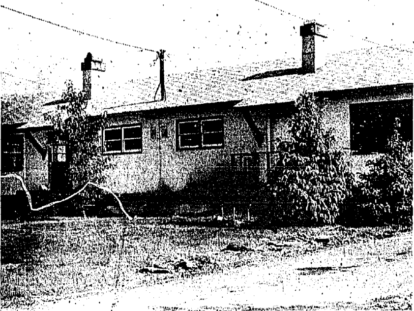
A fire Saturday afternoon in the basement of this house, 38 Lillooet in Kitimat, caused an unestimated amount of damage. The flames spread to the adjacent house, 38 Lillooet, but were controlled by fire officials by about 4 p.m. that same afternoon. Two persons were charged with driving over an unprotected fire hose at the blaze.
