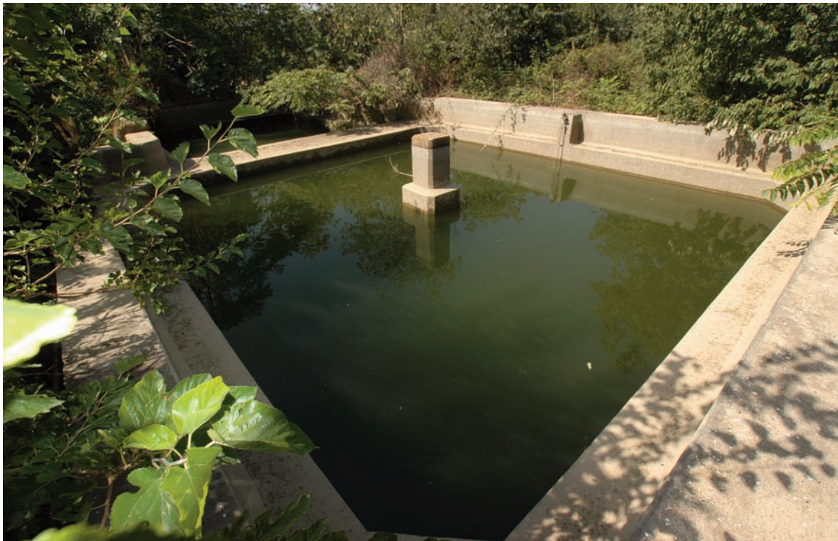
Figure 17. "Ru gebbi" (two gebbie) at Fondo Santacolomba formed by two intercommunicating water tanks.
