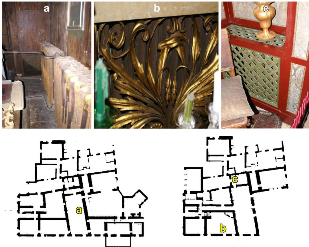
Fig. 3. Location of different radiators and their integration level in the interior design.
